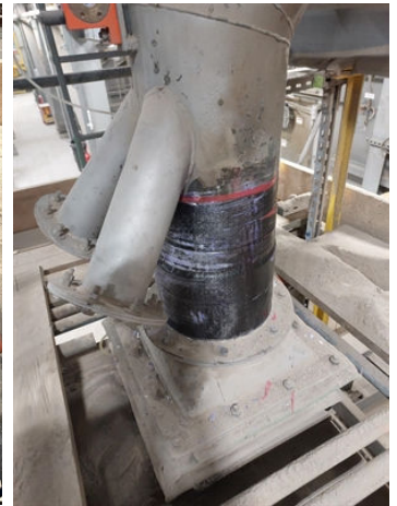
Release film is removed and repair application is complete
