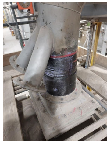
Release film is removed and repair application is complete
