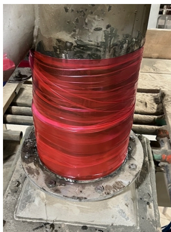
Belzona 1983 SuperWrap II is applied then Belzona 9382 release film is applied to consolidate application
