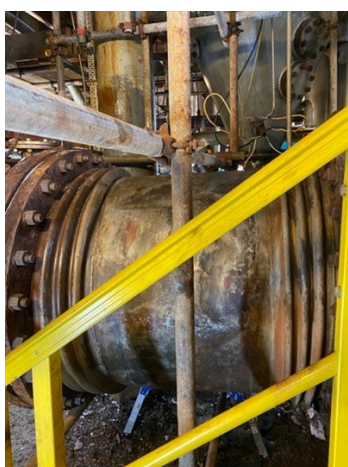
Worn and cracked bellows between two convolutions
