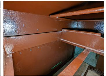
After application of two coats of Belzona 4311.
