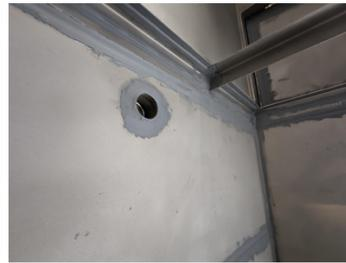
Weld seams and gaps covered with Belzona 1111.
