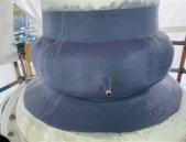
Final application after a further encapsulating layer of Belzona 7311.
