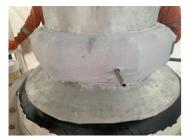
SF6 flange following surface preparation to SSPC-SP11, installation of the Backing Rod, tape, Redirection Nozzle & Breather Membrane.
