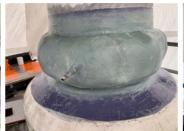
Post-application of 5x wraps of reinforcement sheet (Belzona 9371) and Belzona 1981 resin.
