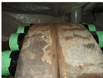
Preparation performed using hand tooling completed.
