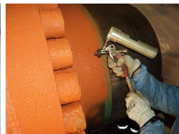
Application of Belzona 3412 encapsulating membrane.
