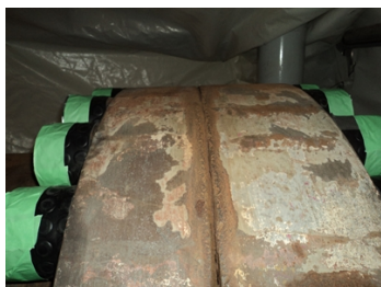
Preparation performed using hand tooling completed.
