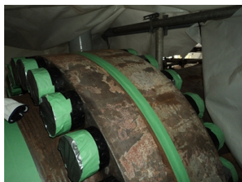
Flanges ready for Belzona 8411 release agent inhibitor.
