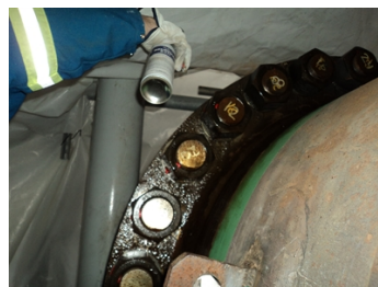
Application of Belzona 8411.
