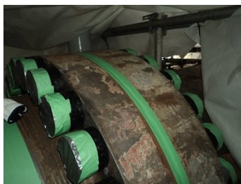
Flanges ready for Belzona 8411 release agent inhibitor.
