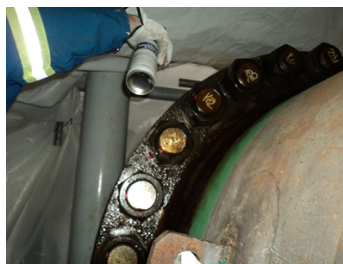
Flanges ready for Belzona 8411 release agent inhibitor.
