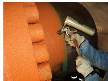
Application of Belzona 3412 encapsulating membrane.
