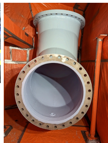
Elbow after application of second coat of Belzona 1341N.
