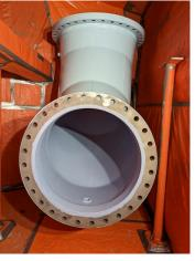
Elbow with deteriorating concrete liner.
