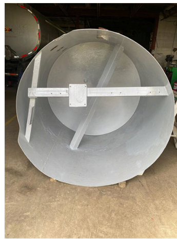
After sand blasting and application of two coats of Belzona 5811
