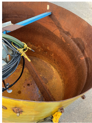
Tank interior prior to application.
