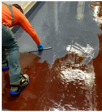
Applying second coat of Belzona 4311
