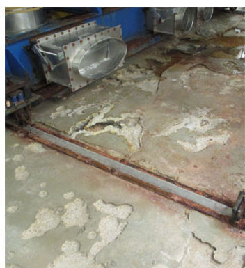
Floor damage caused by Succinic Acid
