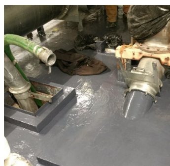
Second coat of Belzona 4311 around floor step up's and piping equipment through floor.
