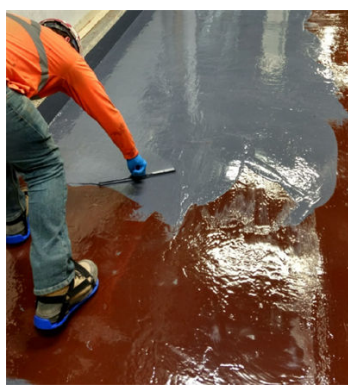
Applying second coat of Belzona 4311
