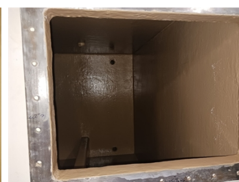
Black Tank After application of two coats of Belzona 5811.
