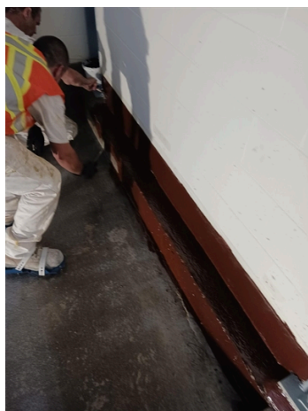
Application of first coat of Belzona 4311
