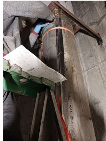
Application of Belzona 1111
