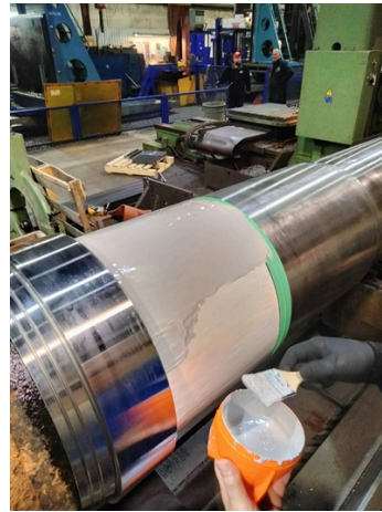
Application of Belzona 1331 second coat
