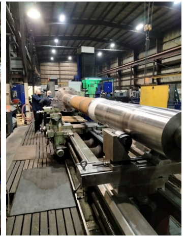
Shaft repair areas waiting on cure times so the machine shop can machine to the correct measurements.
