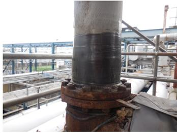
Completed repair with Belzona 1981 SuperWrap 2 installed
