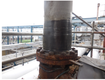
Completed repair with Belzona 1981 SuperWrap 2 installed
