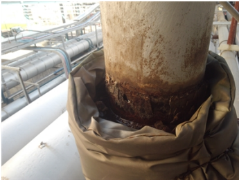
Corroded pipe section
