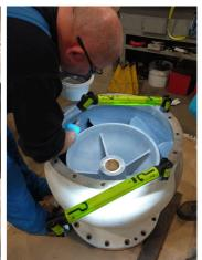
Preparation in progress for Repaired areas of p rebuilding of pumps bowls and using Belzona 1121 suction bell as per the IFU
