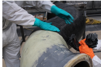
SuperWrap II In progress
