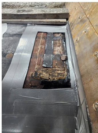
Top layer removed, Belzona 9341 reinforcement sheet pre-cut, border taped off, and Belzona 2911 QD conditioner applied.
