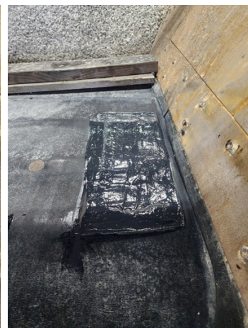
Belzona 2211 application completed.
