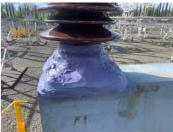
Build up Belzona product, ensuring no air pockets remain. Product given a week to cure before 5 bar restored to the Gas Circuit Breaker
