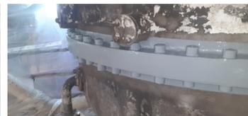
Finally full encapsulation of repairs using Belzona 5811
