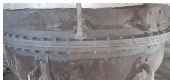
Surface preparation by grit blasting
