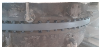
Bolt caps filled with Belzona 1511 and general filling of flange interface.
