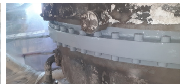
Finally full encapsulation of repairs using Belzona 5811
