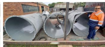
Coating of Cyclones 1 & 2 - showing internal coating completed
