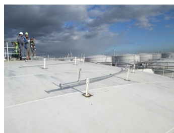
Brackets bonded in place
