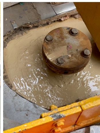
Completion of the application coated with Belzona 5831
