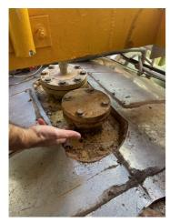
Severe through wall corrosion at the base of the nozzles exposed dangerous chemicals during the process
