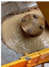
Completion of the application coated with Belzona 5831
