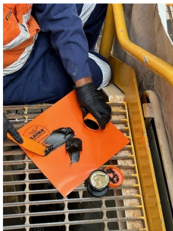
Mixing Belzona 1212 in preparation for the repair
