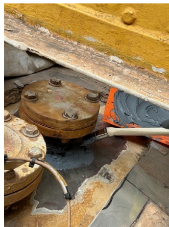
Application of Belzona 1212 over repair area with reinforcement plate/mesh to be fitted
