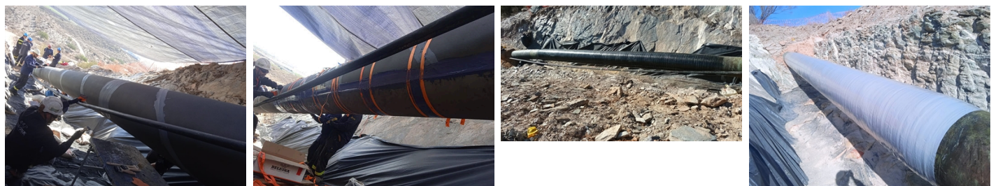
Application start, application of Belzona 1111 to spiral weld area to make a smooth transition Application of Belzona 7311 plate bonds Belzona SuperWrap II system Completed application overcoated with Belzona 5811
