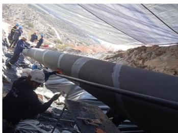
Application start, application of Belzona 1111 to spiral weld area to make a smooth transition
