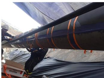
Application of Belzona 7311 plate bonds
