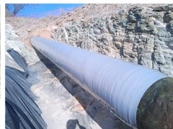
Completed application overcoated with Belzona 5811
