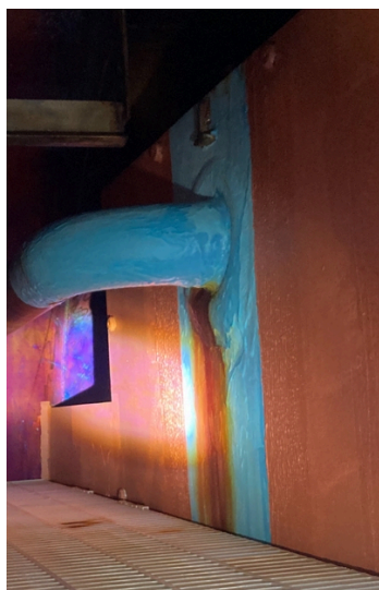
Before the surface preparation
