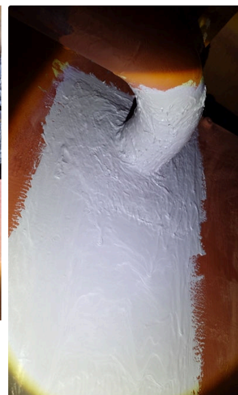
Surface coated with Belzona 1391T
