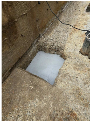
The sump after applying 3 buckets of 4111 to the bottom.
