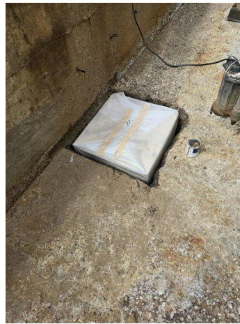
The sump with the plastic wrapped plywood former installed.
