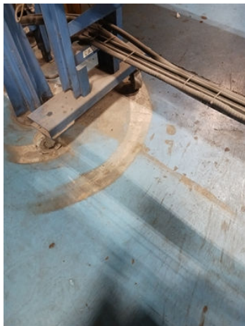
Floor area showing where the grooves have been repaired on this conveyor.
