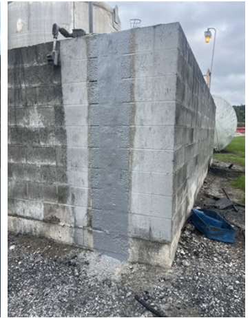
The crack in the outside of wall that was repaired with Belzona and coated
