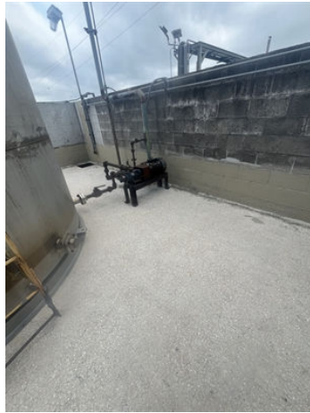
Area after grit blasting
