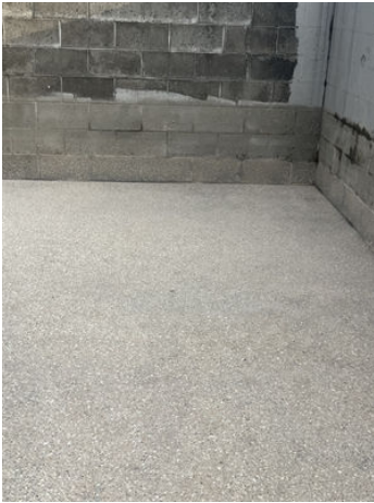
Grit blasting the floor to get correct surface profile.
