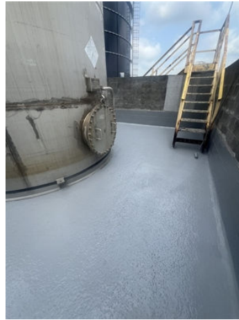
Floor after the second coat
