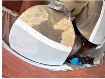
Belzona 1341 grey applied as first coat
