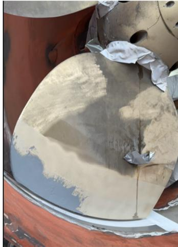
Belzona 1311 applied in areas of cavitation
