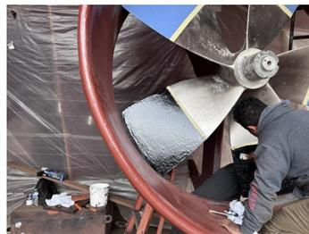
2nd coat applied was Belzona 2141
