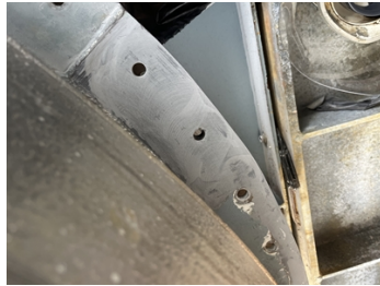
Flange After Repair with Belzona 4301
