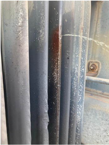
Leaking transformer
