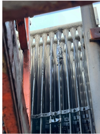
Area completely repaired using the product
