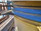
The damaged compensator was finally repaired with the product Belzona 7311.
