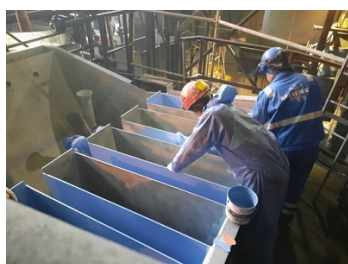
Application of the first layer of Belzona 1341.
