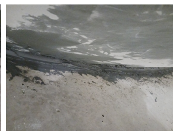
Final sealing with Belzona 1111.
