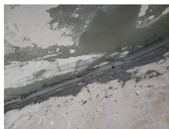
Gap after sealing with Belzona 1111.
