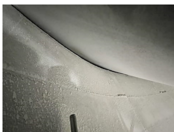
Gap between Silo cone before cleaning
