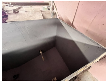
Tank after surface preparation and rebuilding with Belzona 1121.
