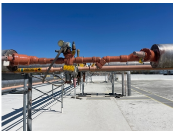
Belzona 5871 applied
