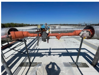
Belzona 5871 applied
