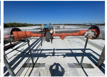
Belzona 5871 applied
