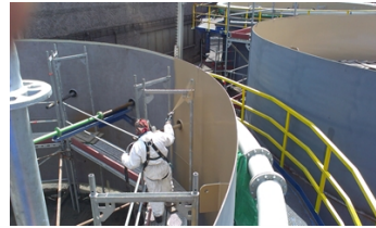
Application of the first layer of Belzona 5811.
