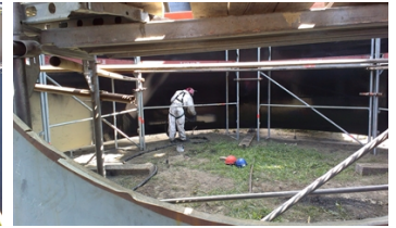
Application of the second layer of Belzona 5811 product.
