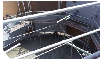
The surface had to be blasted for application.
