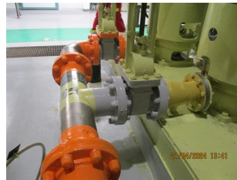
MULTIPLE FLANGES SHOWING FIRST & FINAL COAT APPLICATIONS.
