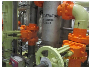
2 X COAT SYSTEM OF BELZONA 3412 PROTECTING FLANGE GASKET AREAS AND FASTENINGS.
