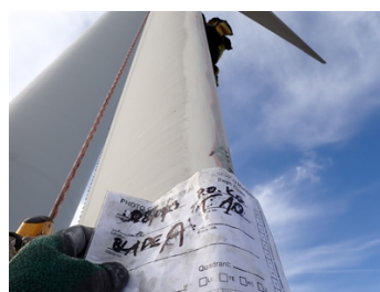
Application of Belzona 5711 and Belzona 5721 completed
