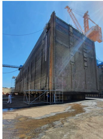
Caisson after the Belzona repair
