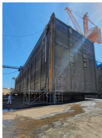
Caisson after the Belzona repair
