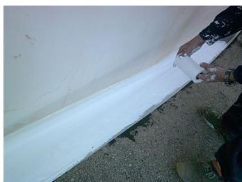
Tank base after the Belzona 3211 application.
