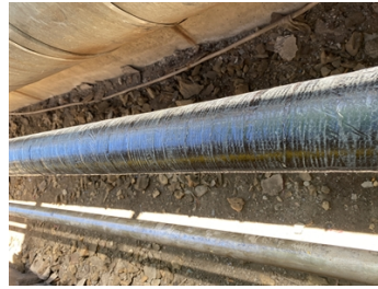
The pipe is encapsulated with Belzona SuperWrap II.
