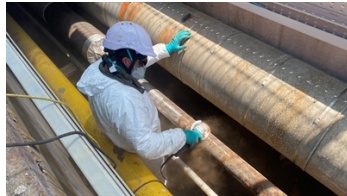
Pipe during surface preparation.
