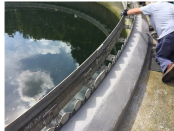
Applying Belzona 4131
