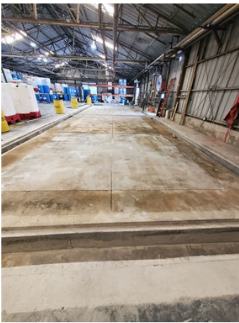
New uncoated containment area
