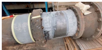
The pipe after being repaired with Belzona 1121.
