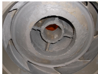
Belzona 1111 filling in all of the damage and correcting the profile.
