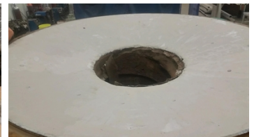
Belzona 4111 application complete.
