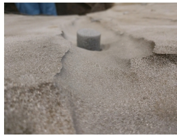
Backer rods inserted into the wear plate mounting holes and showing the target profile height.
