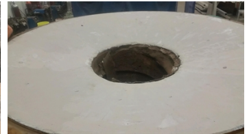
Belzona 4111 application complete.
