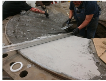
Applying Belzona 4911 Conditioner in the background, and applying Belzona 4111 using a guide to achieve the proper profile.
