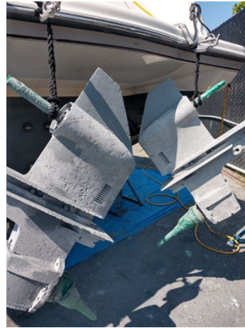
Belzona 1111 being applied to rebuild the missing material and smooth over the pitting.
