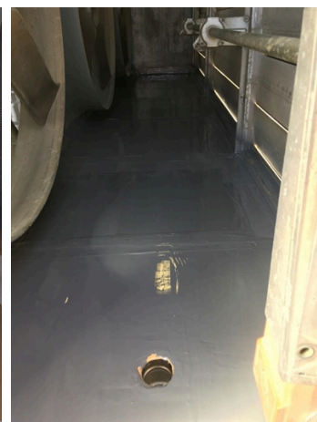
Second coat of Belzona 5831 applied, application complete.
