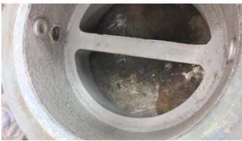
Check valve grit blasted and ready for application.
