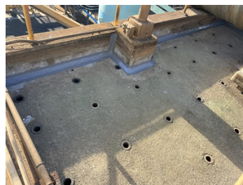
Belzona 3121 Applied with Reinforcement Cloth
