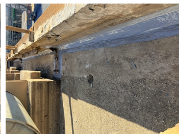
Belzona 3121 Completed
